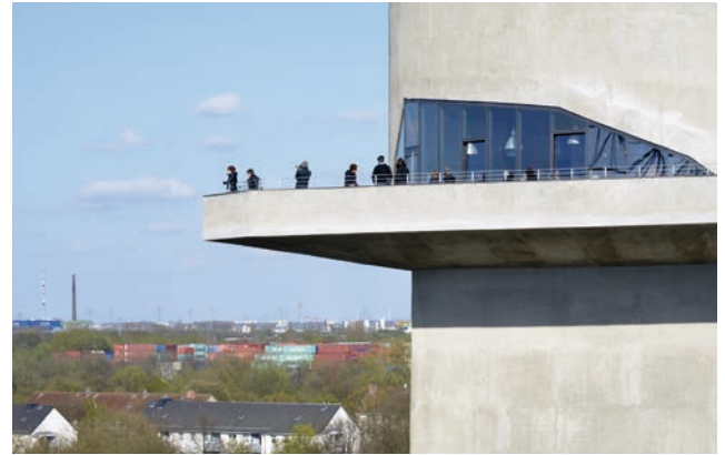
Energiebunker in Hamburg-Wilhelmsburg
